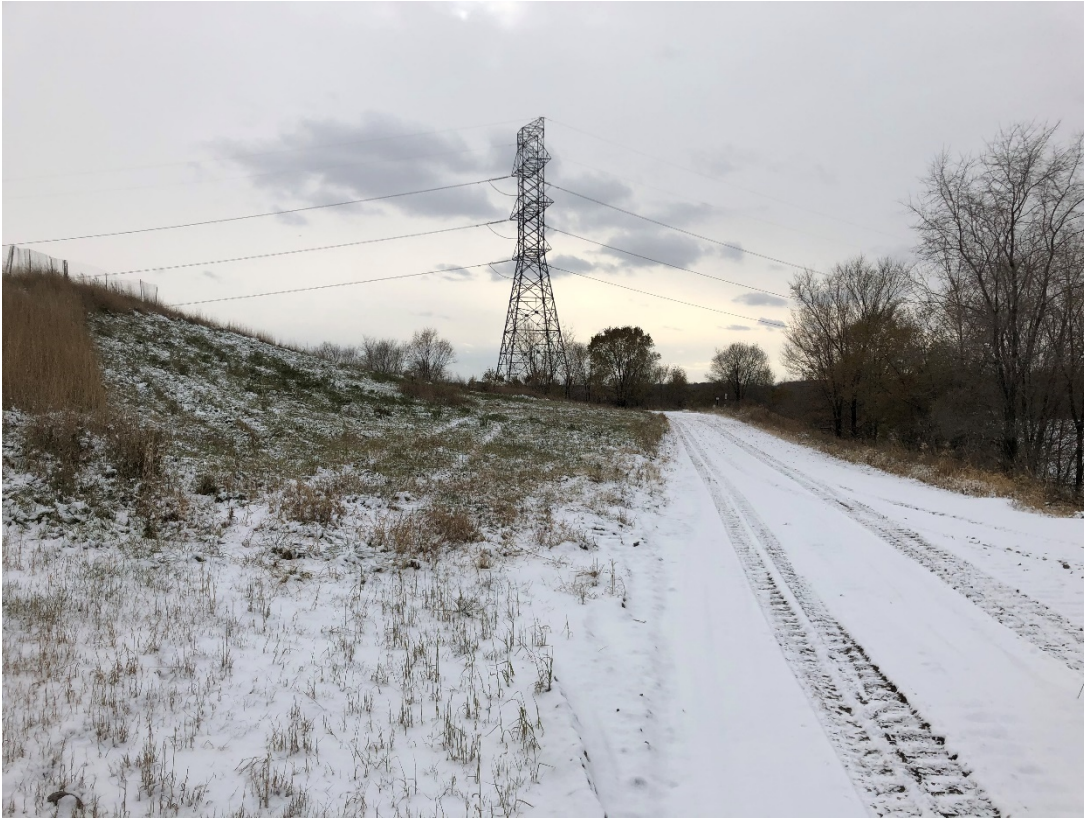
Photo 35: Location 12 – Looking Southwest, Cell 2A Northwester Waste Slope and Anchor Trench
