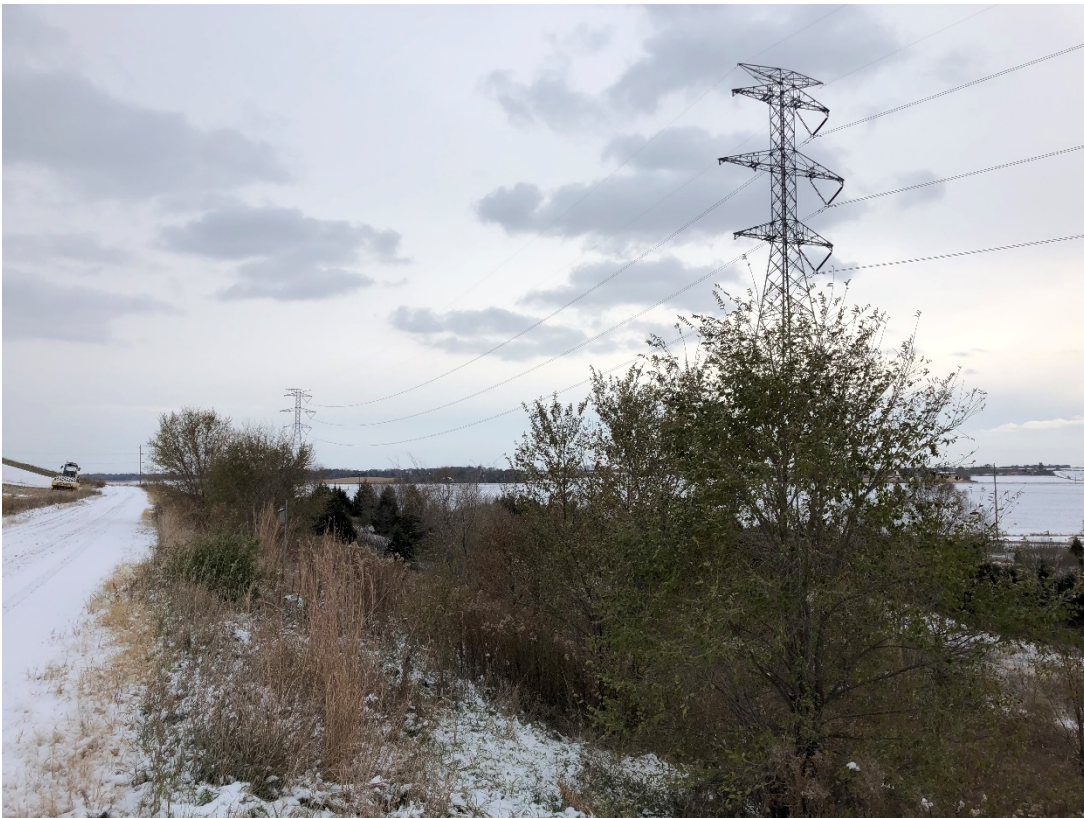
Photo 16: Location 7 – Looking Southeast, Cell 2D Berm
