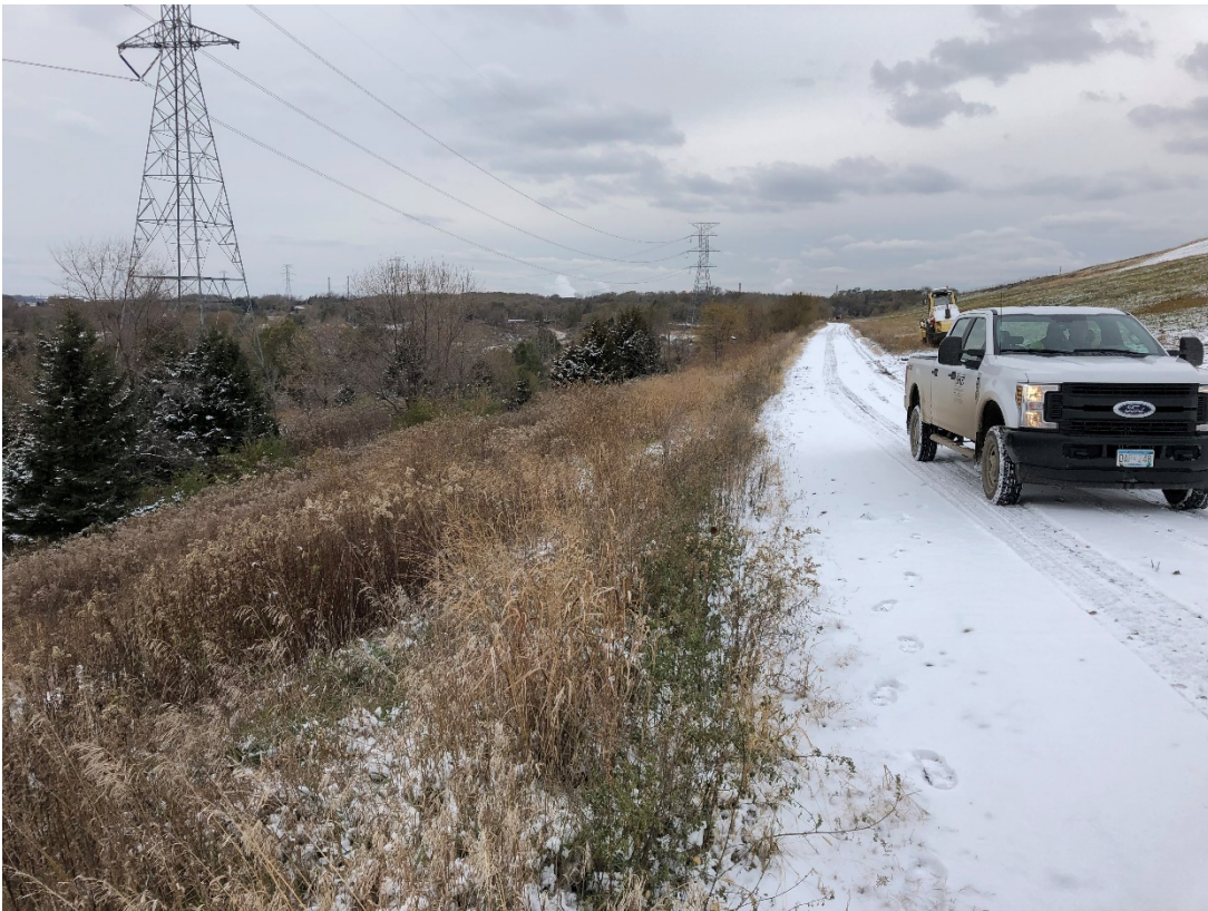
Photo 14: Location 6 – Looking North, Cell 2D Berm
