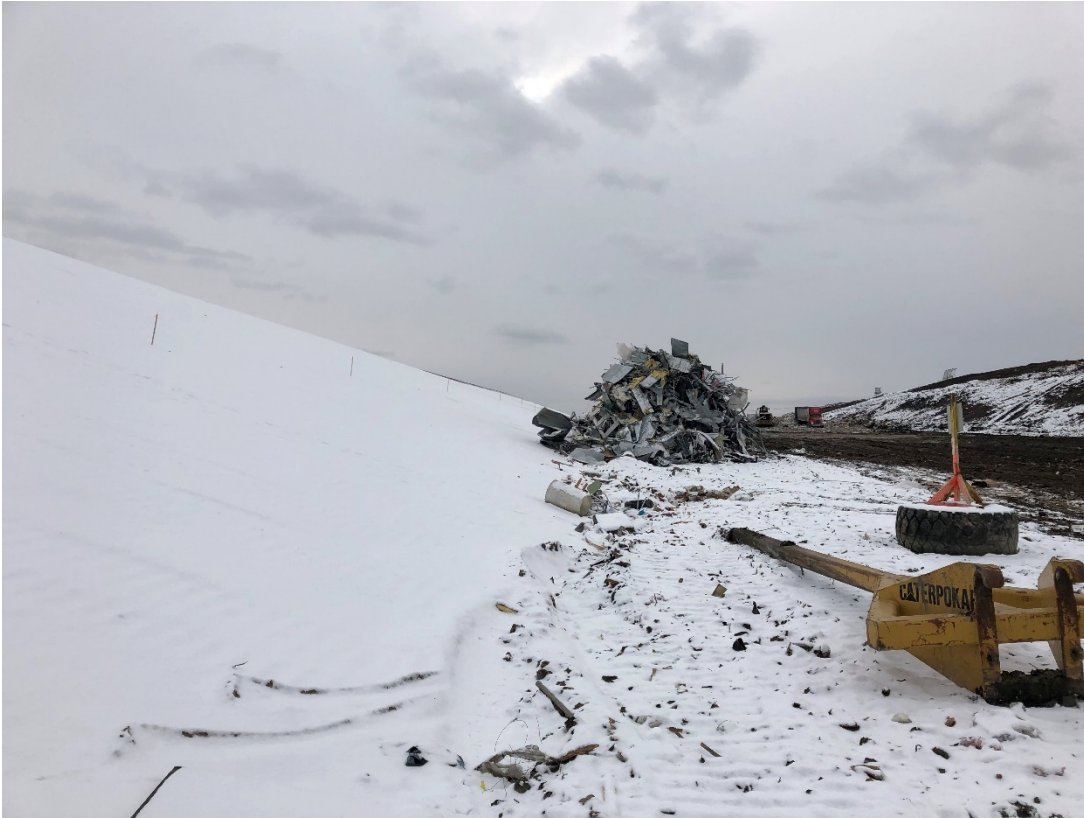
Photo 9: Location 4 – Looking Southwest, Phase 3F Liner Limit
