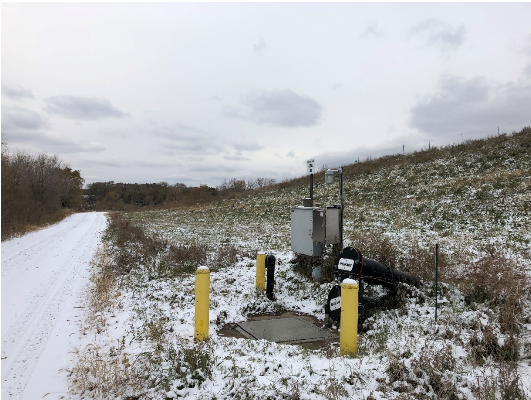
Photo 28: Location 10 – Looking Northwest, Cell 2A Southwestern Waste Slope and Perimeter Road
