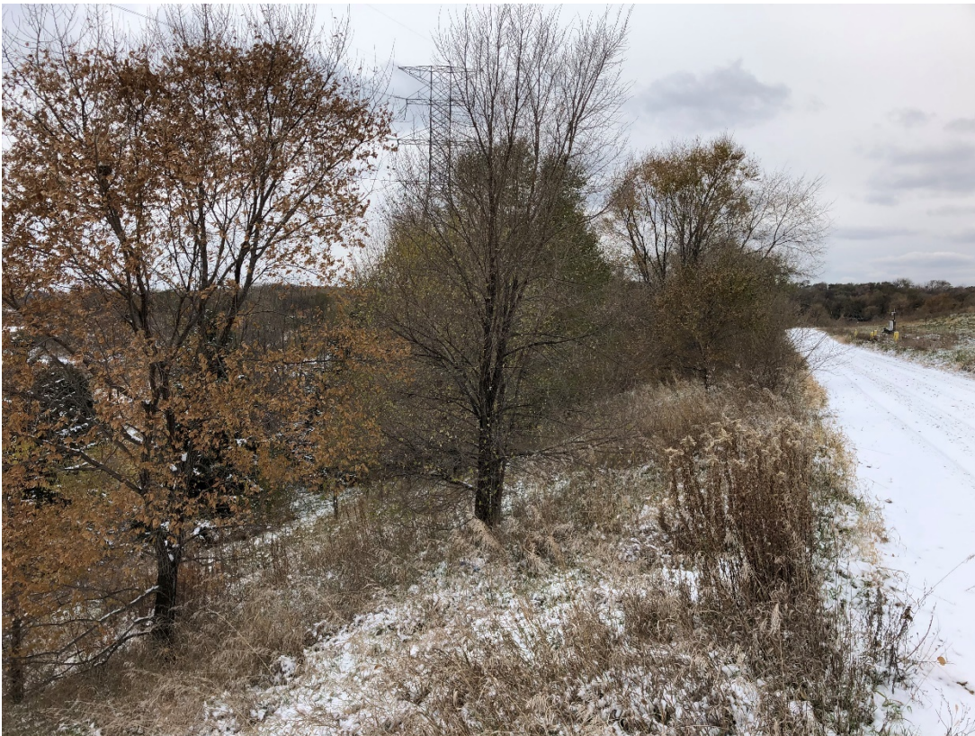
Photo 26: Location 10 – Looking Northwest, Cell 2A Southwestern Berm
