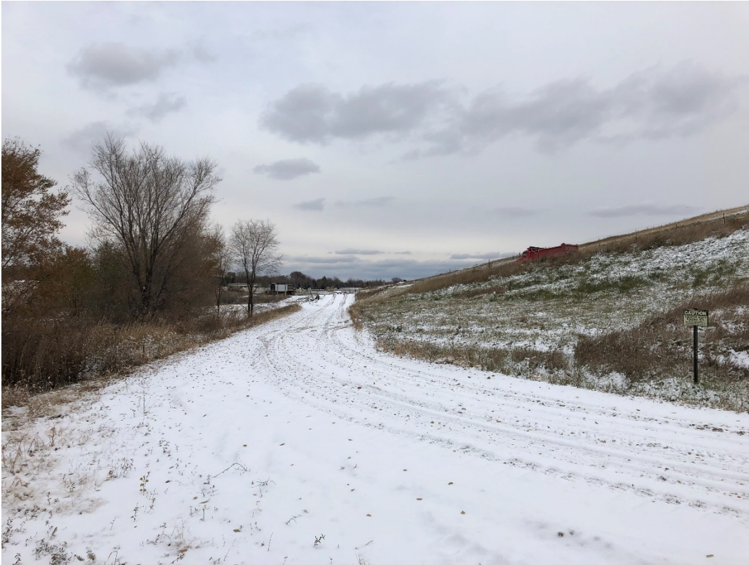
Photo 33: Location 11 – Looking Northeast, Cell 2A Northwestern Perimeter Road and Anchor Trench
