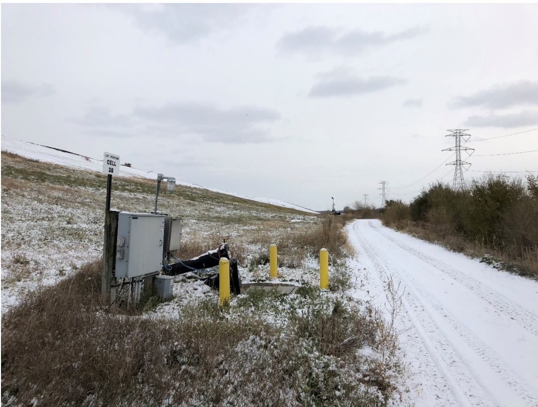
Photo 22: Location 9 – Looking Southeast, Cell 2C Southwestern Waste Slope and Anchor Trench
