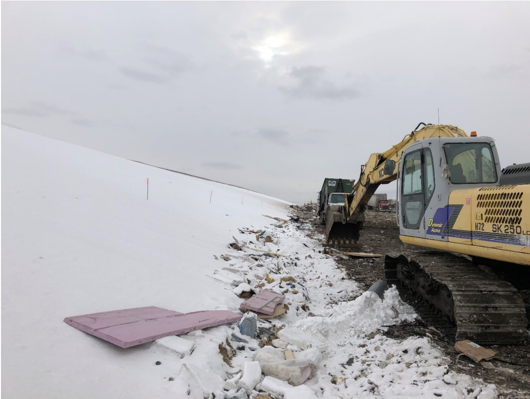
Photo 11: Location 5 – Looking Southwest, Phase 3F Liner Limit
