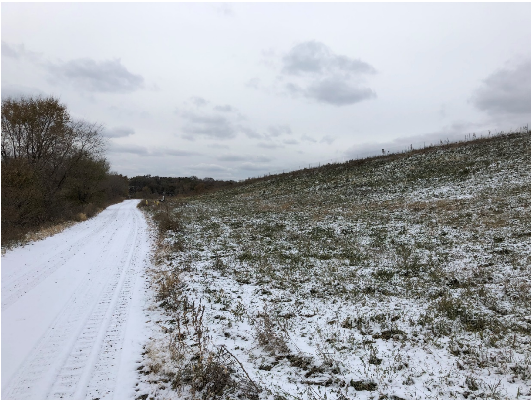
Photo 24: Location 9 – Looking Northwest, Cell 2B Southwestern Waste Slope and Anchor Trench
