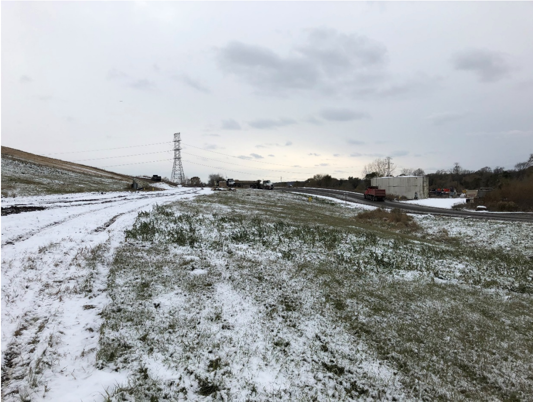
Photo 37: Location 13 – Looking Southwest, Cell 1 Northwestern Berm
