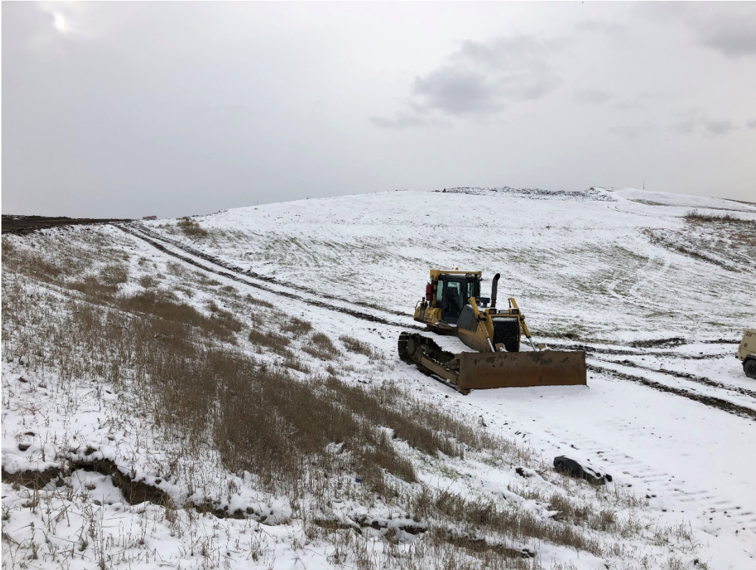
Photo 7: Location 3 – Looking West, Phase 3 East Corner & Interior Access Road
