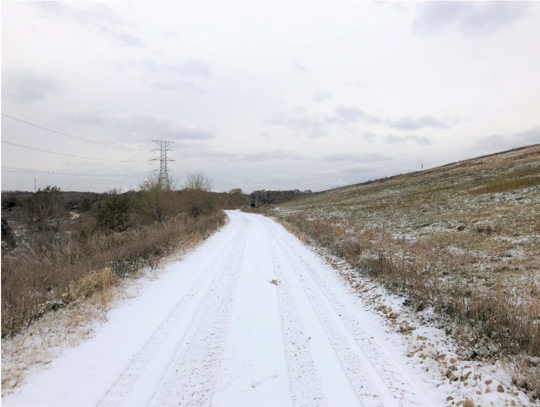
Photo 17: Location 7 – Looking Northwest, Cell 2C Southwestern Slope, Anchor Trench, and Road
