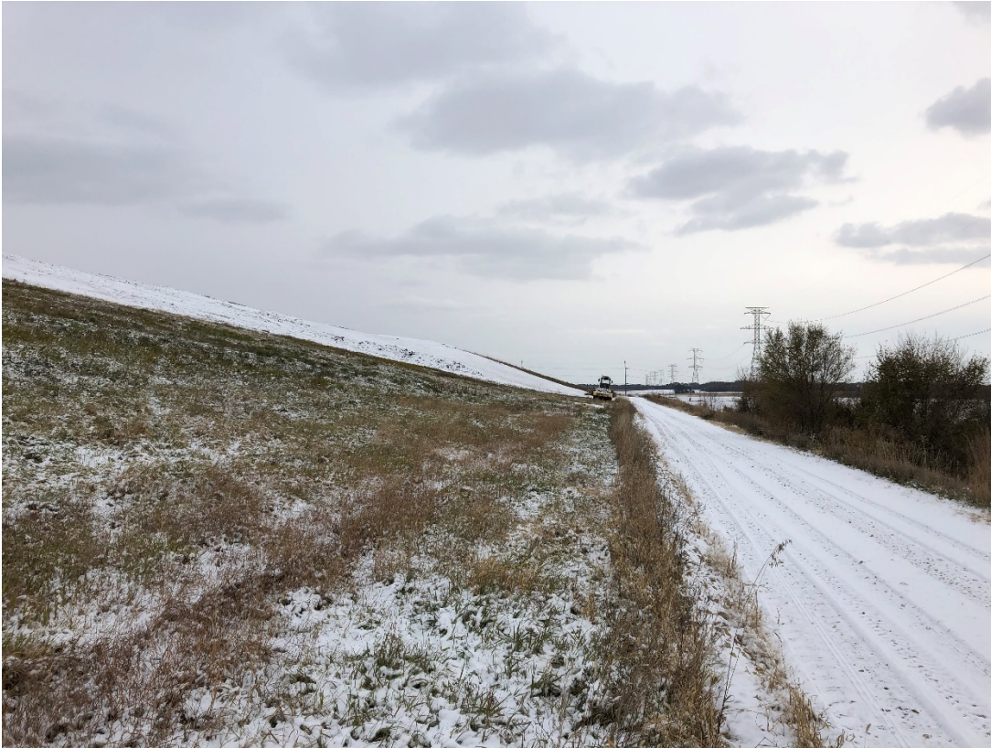
Photo 15: Location 7 – Looking Southeast, Cell 2D Southwestern Slope, Anchor Trench, and Road
