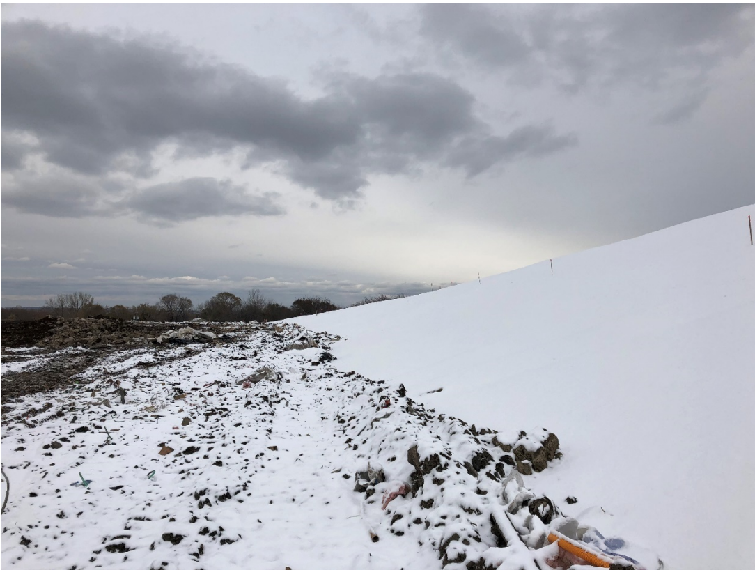
Photo 8: Location 4 – Looking Northeast, Phase 3F Liner Limit
