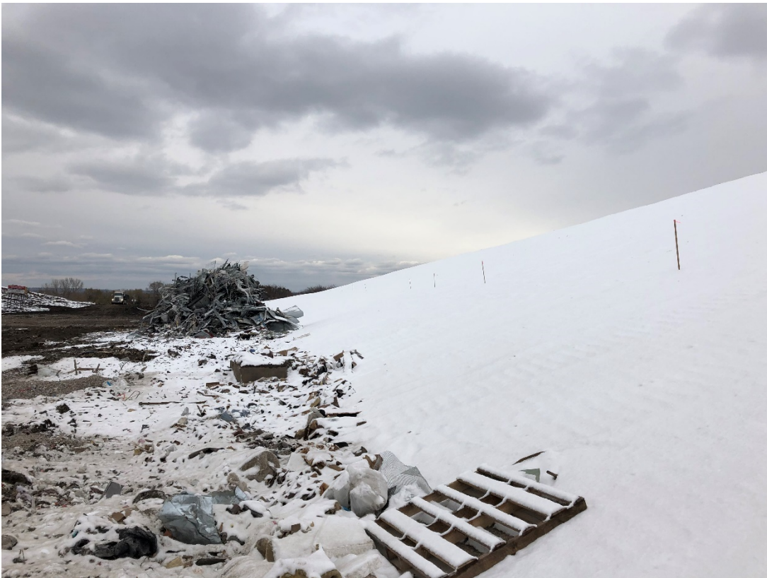
Photo 10: Location 5 – Looking Southwest, Phase 3F Liner Limit
