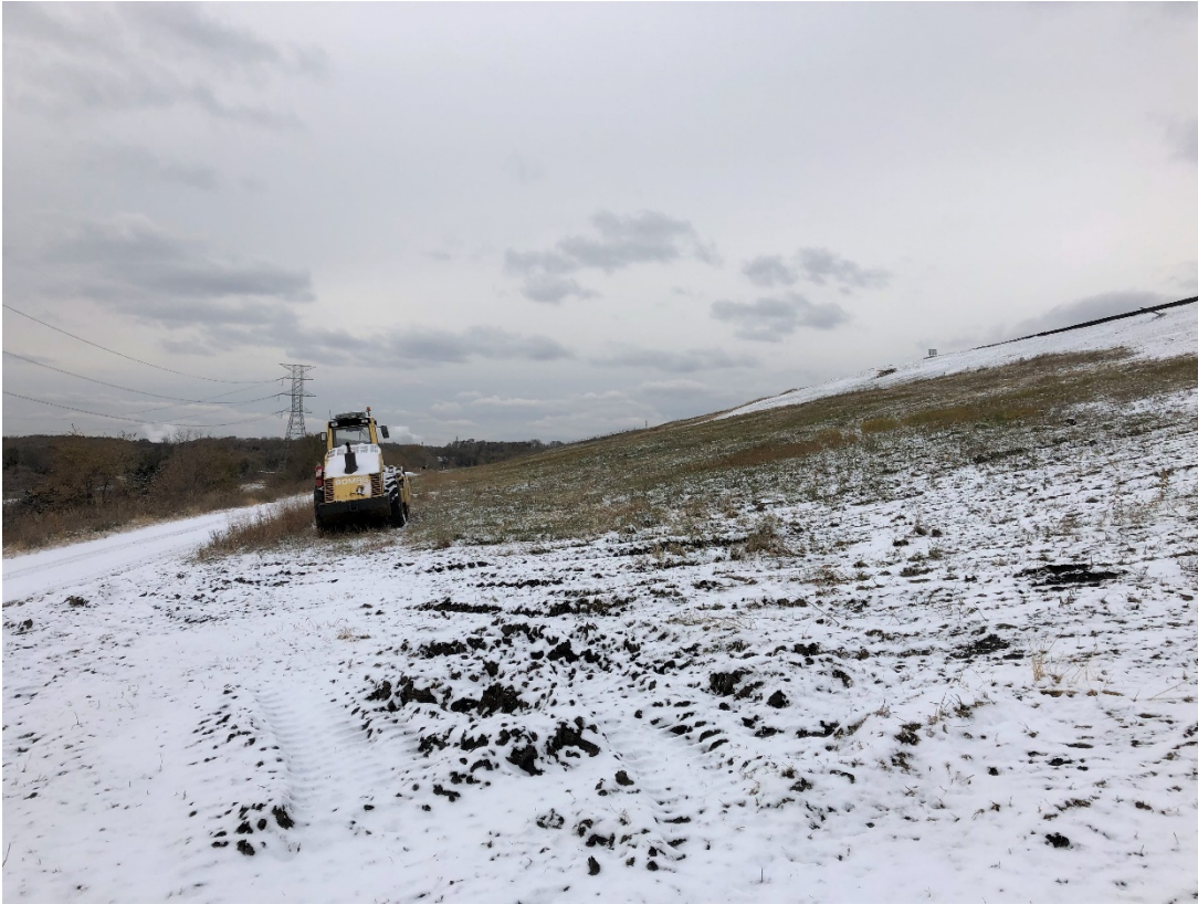
Photo 13: Location 6 – Looking Northwest, Cell 2D Southwestern Slope and Perimeter Road
