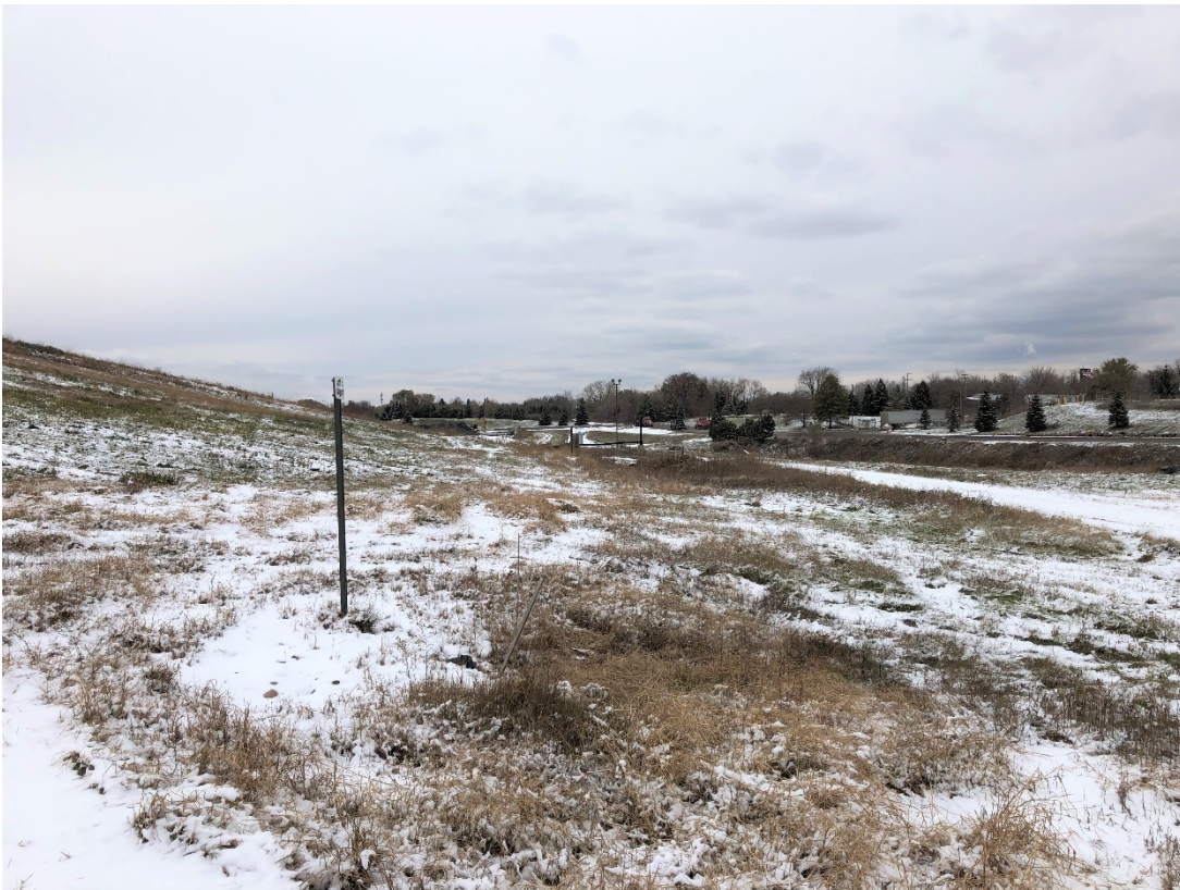
Photo 2: Location 1 – Looking Northwest, Cell 3 Berm
