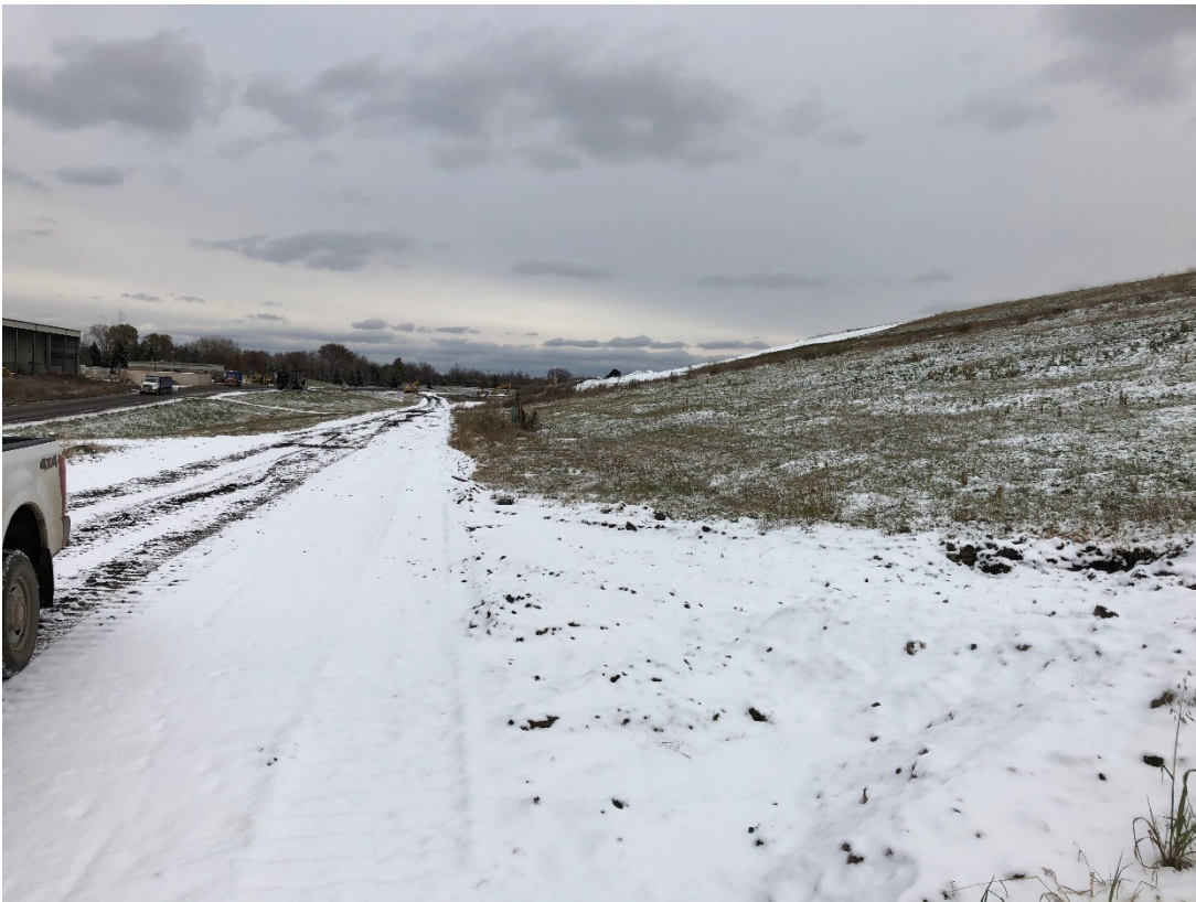
Photo 36: Location 12 – Looking Northeast, Cell 1 Northwestern Waste Slope
