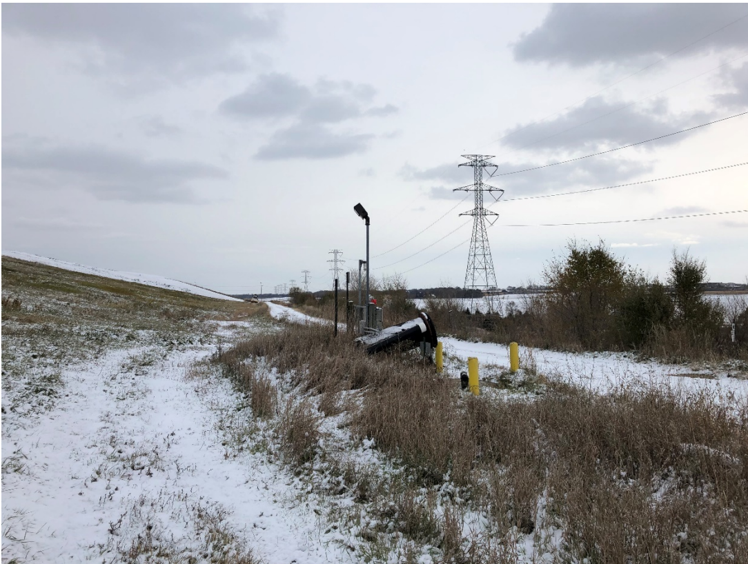
Photo 20: Location 8 – Looking Southwest, Cell 2C Southwestern Waste Slope and Anchor Trench
