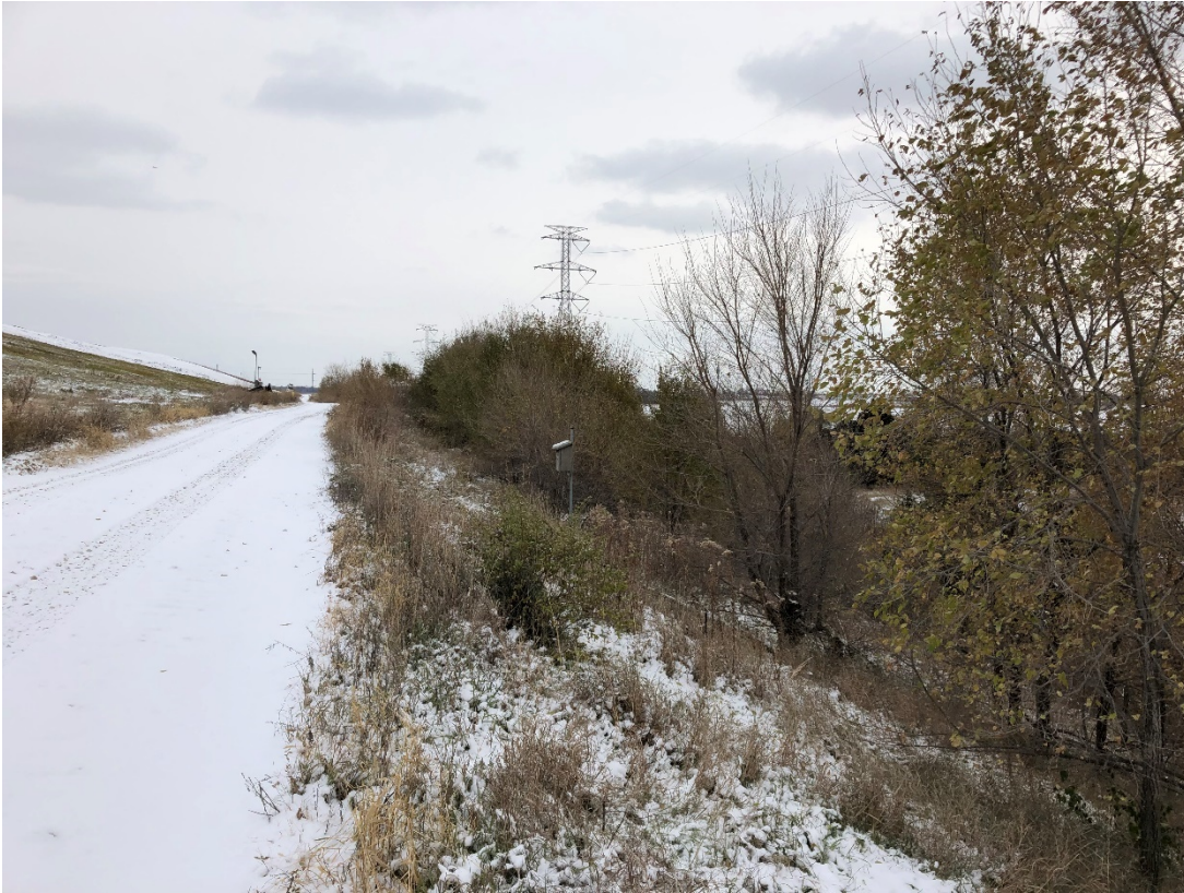
Photo 23: Location 9 – Looking Southeast, Cell 2C Southwestern Berm
