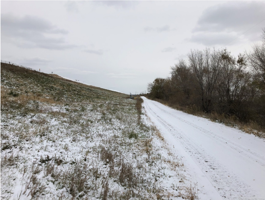
Photo 31: Location 11 – Looking Southeast, Cell 2A Southwestern Waste Slope
