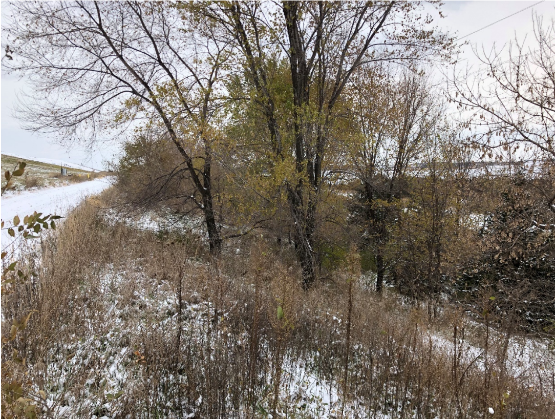
Photo 27: Location 10 – Looking Southeast, Cell 2B Southwestern Berm
