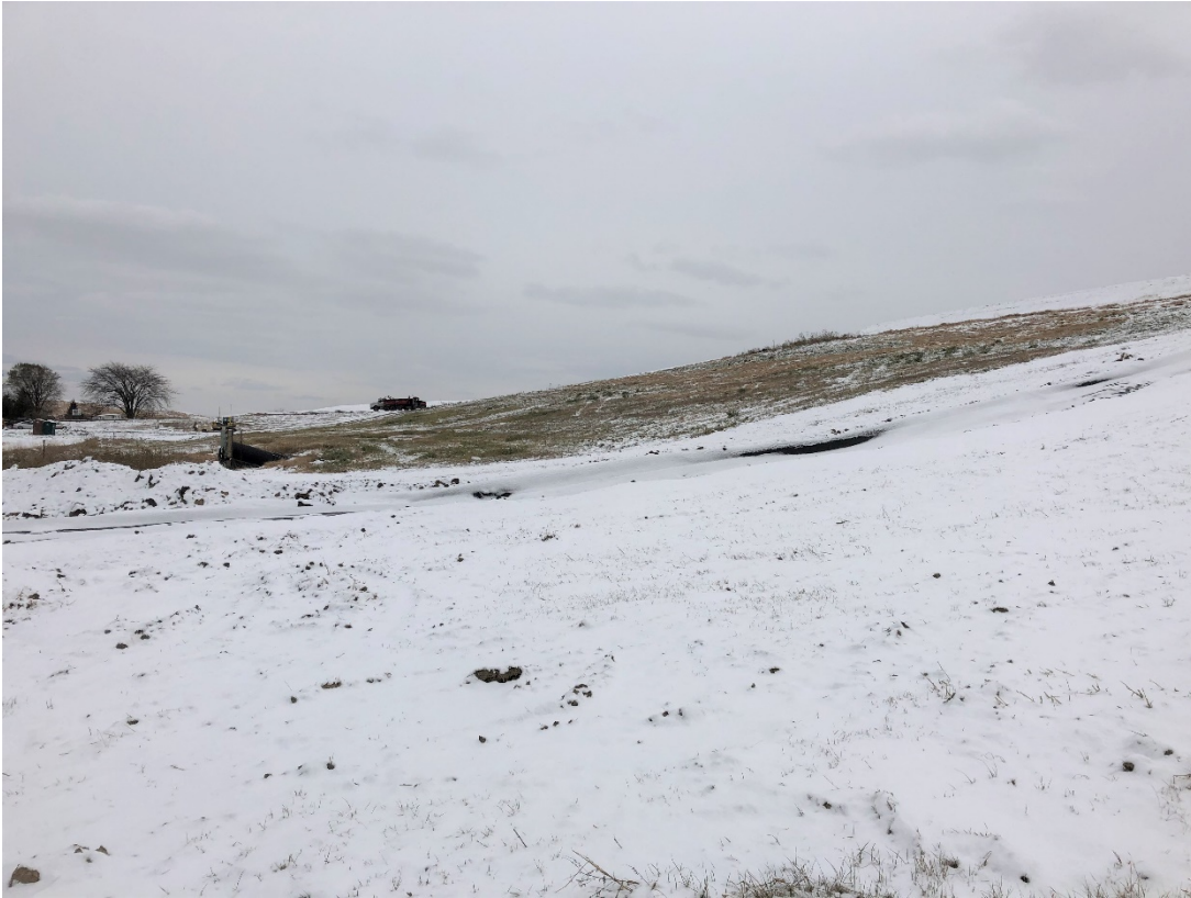
Photo 1: Location 1 – Looking Southeast, Cell 3A & 3B Waste Slope & Anchor Trench
