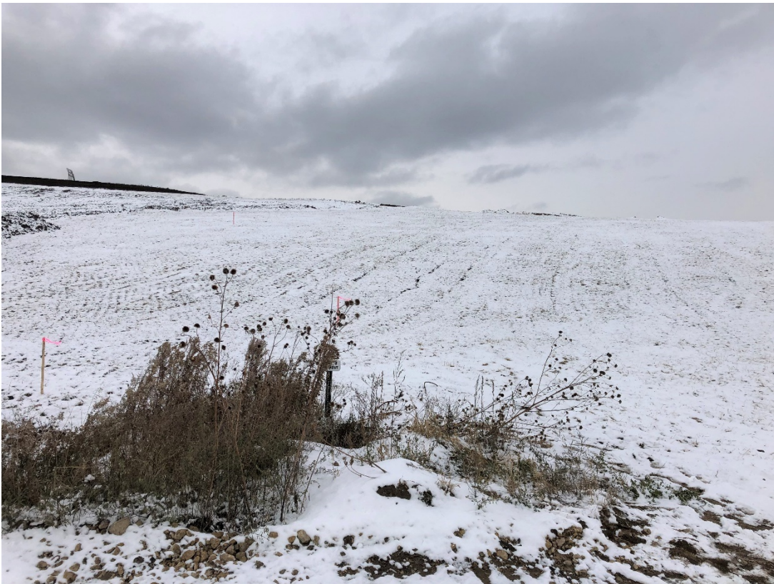
Photo 12: Location 6 – Looking Northeast, Southeastern Slope, Anchor Trench & New Liner Construction
